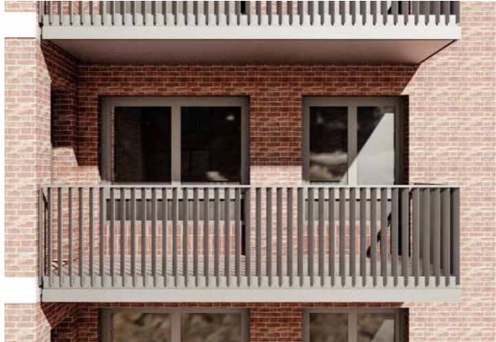
02a Woodberry Down balconies
