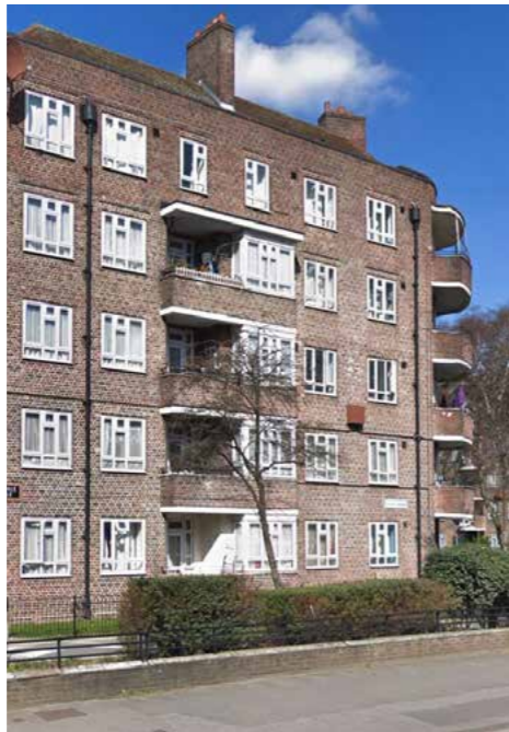
04 phase 6 stacked balconies
