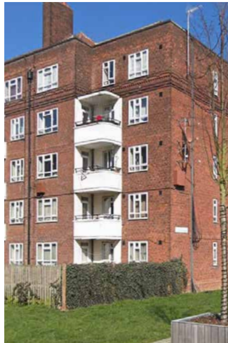
05 phase 4 corner balconies
